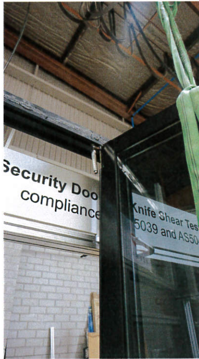
Figure 6: Damage to the top hinge after pull
