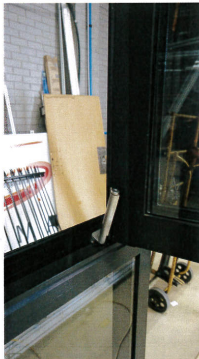
Figure 7: Damage to the bottom hinge after pull
